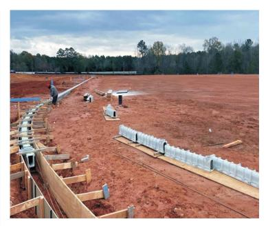
These features helped save the team time and labor and made for an easier installation process compared to competitive products. In addition, construction covers were included on the material to help keep the channels clean and ready for the grate installation when construction was complete.
